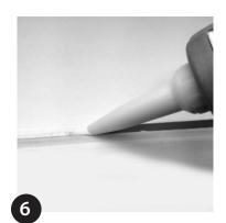
Using appropriate filling material (grout, silicone or mortar) fill down the edges of the GROOVE Light IP67 product into the recessed channel. Ensure that a fair amount of filling material is pushed down the sides of the product and channel to ensure good adhesion.
