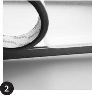
It is advised to mask the front edge of the GROOVE Light IP67 product to ensure that the face of the product is not marked during installation.
