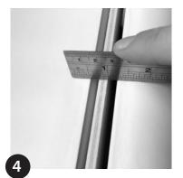
Fit the masked GROOVE Light IP67 into the channel taking care to set the product to the correct depth with relation to the channel.
