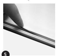
With the GROOVE Light IP67 pushed into the mounting channel, make wiring connections and conceal wiring into recessed channel as required.
