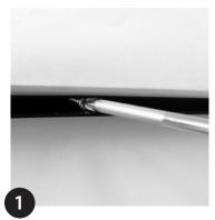
PVC Channel should be secured using suitable fixings for the mounting surface. The PVC Channel can be used to support the entire GROOVE Light IP67 length (Channel length = fitting length), or cut into smaller sections. Minimum 200mm (7.87") of PVC Channel recommended per 500mm (19.69") of GROOVE Light IP67.
